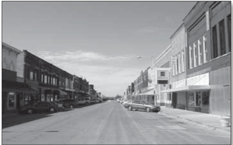
Belle Plaine's main street business district as it looked in 2005 before rehabilitation began.
