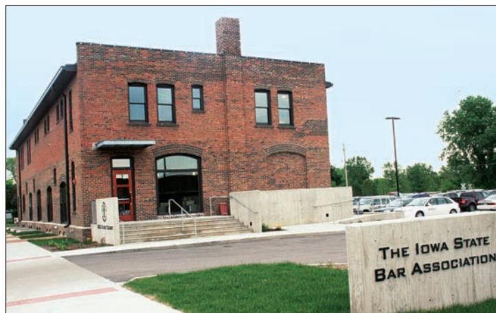
The front of the completed ISBA building from 6th Street and Court Ave., downtown Des Moines, Iowa.
